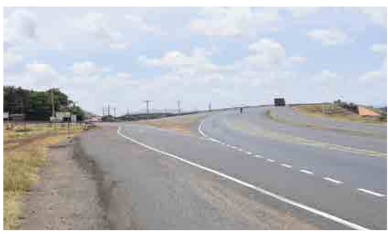
Figure 14: Unsafe configuration at Emali/Oloitoktok Junction
