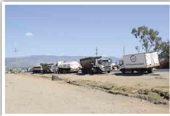
Figure 25: Heavy trucks parked on the shoulders effectively narrowing the carriageway and impairing visibility for other road users
