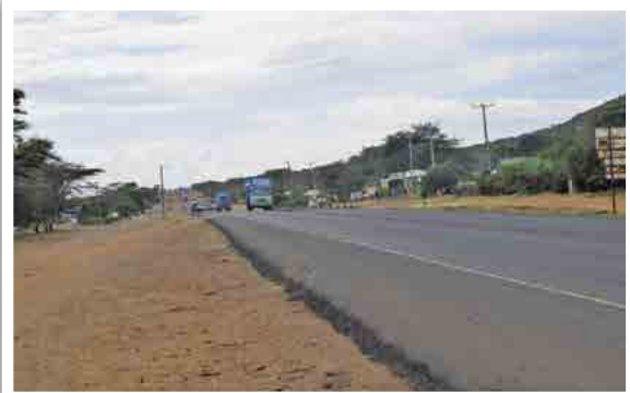
Figure 17: Kalimbini area (Long and straight stretch with a slight descent from the Nairobi side prompting motorists to overspeed and overtake recklessly)
