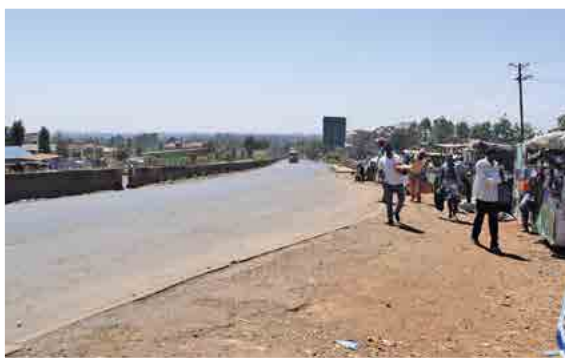
Figure 20: Encroachment of the road reserve by vendors/hawkers
