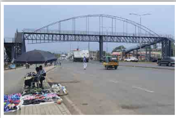
Figure 33: Pedestrian dangerously crossing the highway at grade despite provision of a footbridge
