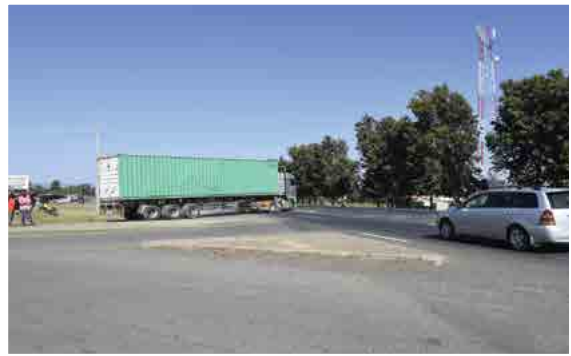
Figure 22: Heavy truck joining the A8 Highway from Njoro (note the narrow turning radius).
