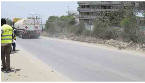
Figure 2: Missing road markings at Makupa Causeway
