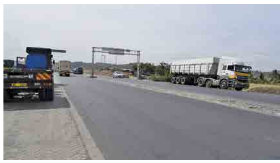
Figure 8: Faded road markings
